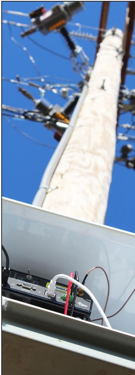
The fiber network is allowing us to extend the SCADA system to breakers in the field.
